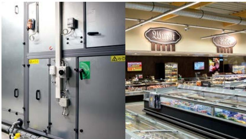
The remaining heating is managed by an add-on heating register, which is fed with the waste heat of the supermarket's freezers. If the market has to be cooled, the  $Ka_2O$  technology activates and transmits almost 100 % of the wet bulb temperature of the extract air to the outside air.
