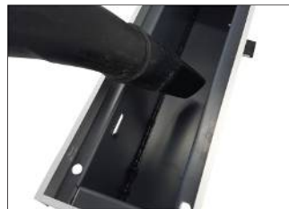
▶ Vacuum or wipe the floor trench.
